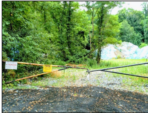
Figure 1. Project Work Site - Leone Pit (Area L) gate. The soil seen here beneath tarps will be removed during hunting season.
