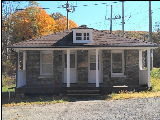
Figure 1. Bldg 1666 - AKA the Snake Pit - as of 2022, the new Hunt Control and Harvest Check Station site.
